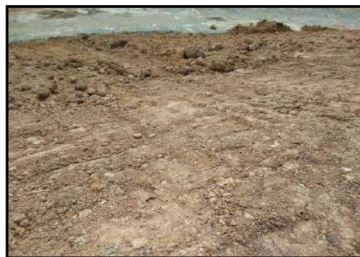
Gambar 4.5 Penebaran Tanah Pucuk ( Top Soil )
